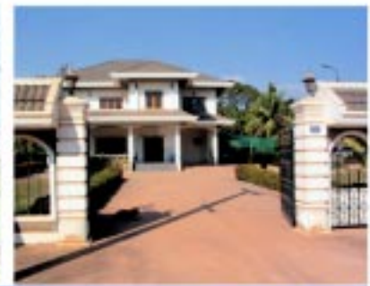
Colonial style gates and fences
