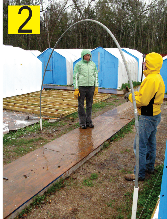
Testing the first arch for vertical clearance
