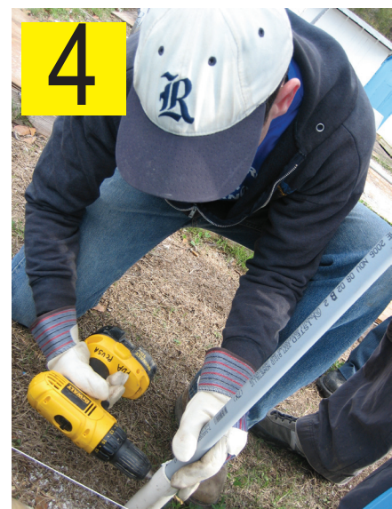
Attaching the PVC pipe and conduit together with zip ties
