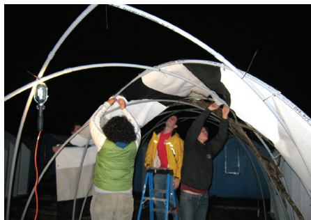
Fixing fabric to frame
