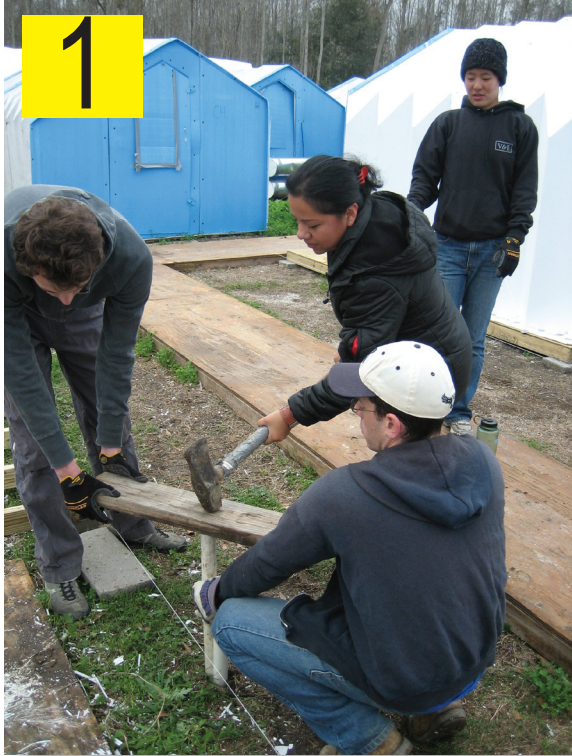
Driving the PVC pipe into the ground
