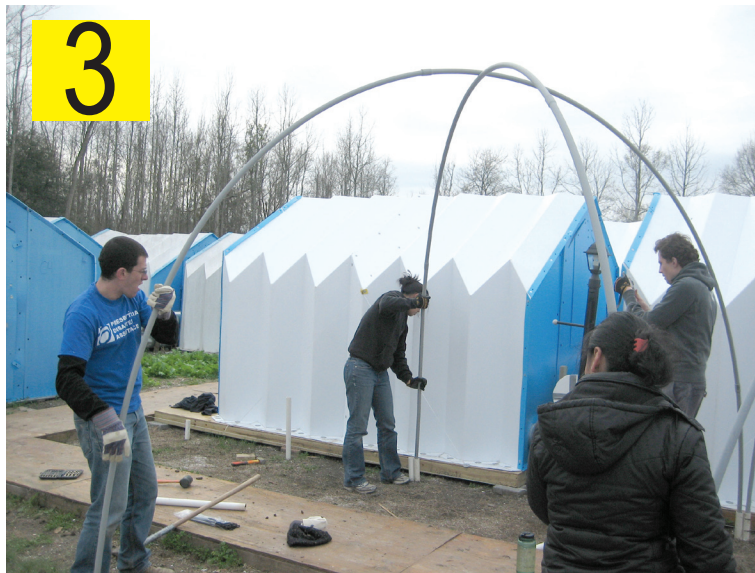
Assembling the arches
