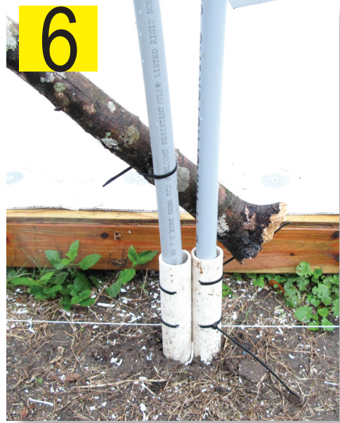
Detail of arch base with zip tie attachment of PVC pieces and wood ornamentation
